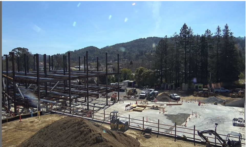
Learning Resources Center Steel Erection, Kentfield Campus
